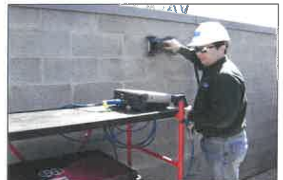
Surface Penetration Radar Scan on Concrete Masonry
