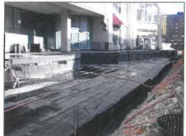
Plaza hardscape demolition and new continuous, fluid-applied waterproofing
